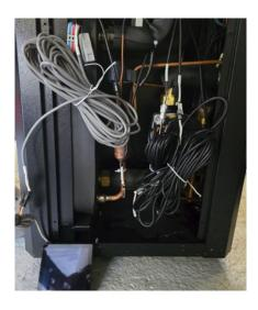
The controller plugs into the unit using a black plug on a grey cable. It has a 10 m grey extension cable. The controller needs to be installed inside the property in a heated space. Note the plug on the controller wire is 16 mm across so you will need to drill 16 mm holes to get this into the house.
