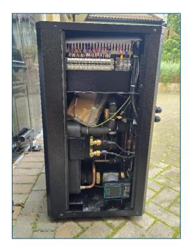
A power supply is needed at the outdoor unit. A 32 Amp Isolator is provided in the Heat Pump Accessory Kit. It must be within 1 m of the unit.
