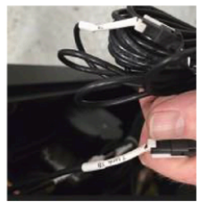
Room thermostats wire from 4 to 5, unit runs in heating when link is made.
